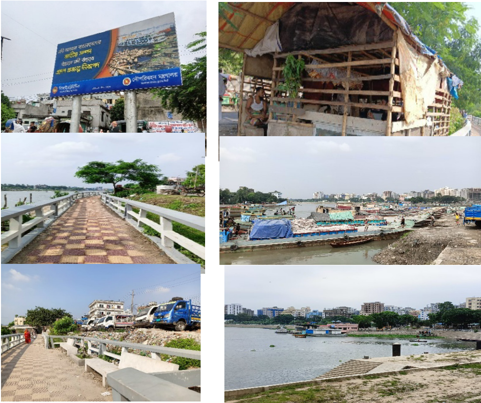
Figure 4 Existing facilities at the waterfront
